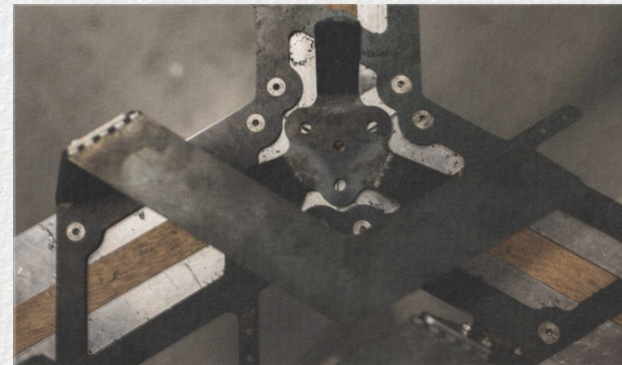
◀ Unit 8 Show detail (2016) 2mm Steel junction plate secured directly to aluminium extrusion with M4 countersunk machine screws.
